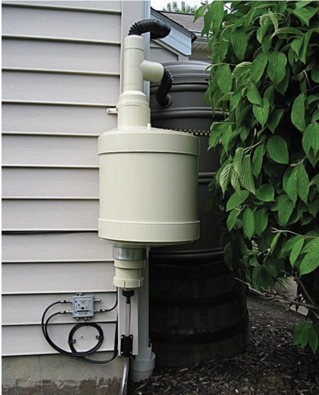
Left: The assembled diverter, after spray painting to match the house. Ignore the wiring, it is unrelated. Right: Two rainwater collection barrels are now full of clean, clear water, thanks to the working diverter.
