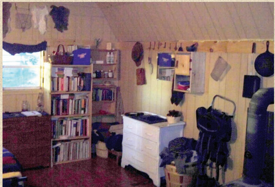
The taller side walls of the larger storage barn were insulated and covered with inexpensive birch paneling. Additional insulation went into the ceiling.
