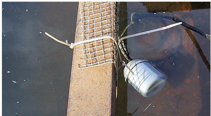
Float switch used to shut off pump when the tank is full to prevent overflow which can muddy ground and waste water
