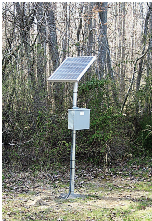
Pole-mounted solar module and pump controller next to drilled well
